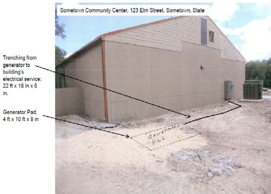
Figure 4. Ground-level photograph showing proposed ground disturbance area.
